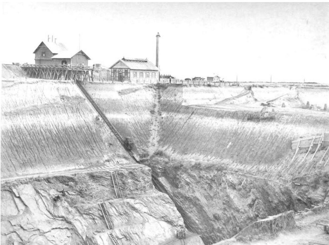
Fig. 2. Open-pit iron mine near Krivoy Rog taken by an unknown photographer circa 1900. Approximately 25 m of sediments (massive, unconsolidated, rilled) overlie steeply dipping schistose units of the Precambrian Shield. The terrace at the top of the uppermost ladder marks the interface between overburden and crystalline rocks.
